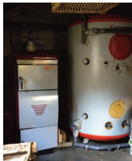
Angus Orligno 200 40kW log batch boiler & 1500L thermal store.
