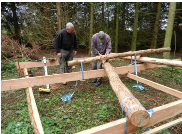
The framing bed with joints being marked up.
