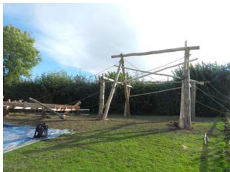
A frames with Jowl posts and cross bracing added.
