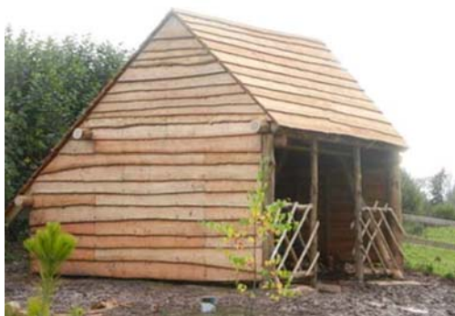
The front timbers are peeled Ash.
